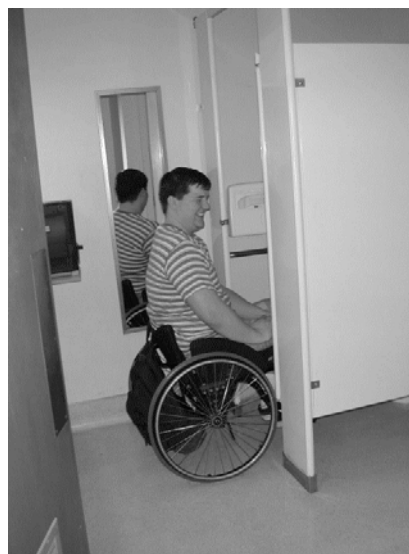
Figure 6.16: Wheelchair user unable to pass through men's toilet stall door.
