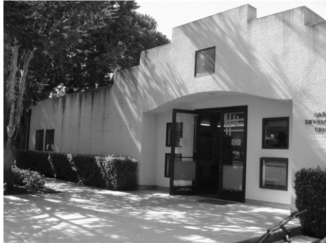
Figure 6.2: CDC entrance close-up.
