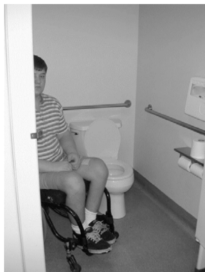
Figure 6.12: Wheelchair user access to the women's toilet.
