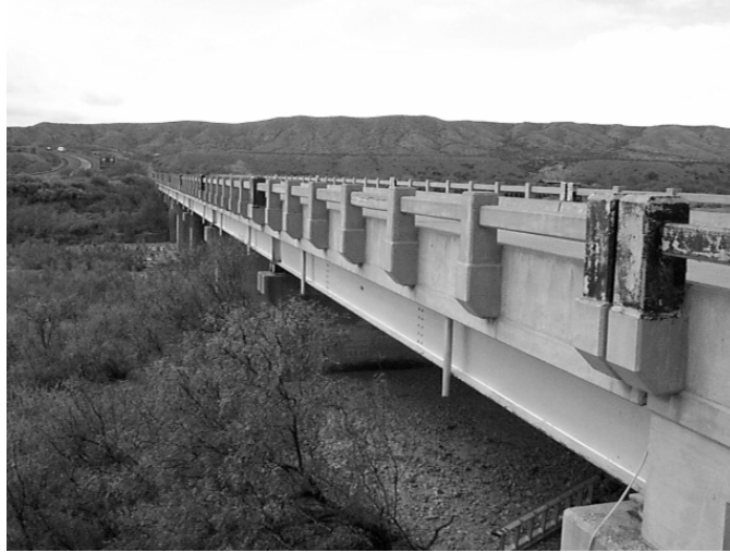
Figure 1. A Side View of The Alamosa Canyon Bridge
