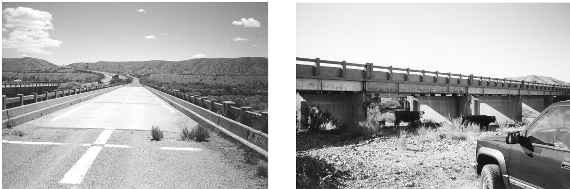
Figure 4: Views of the Alamosa Canyon Bridge: (left) top roadway looking south and (right) side view
