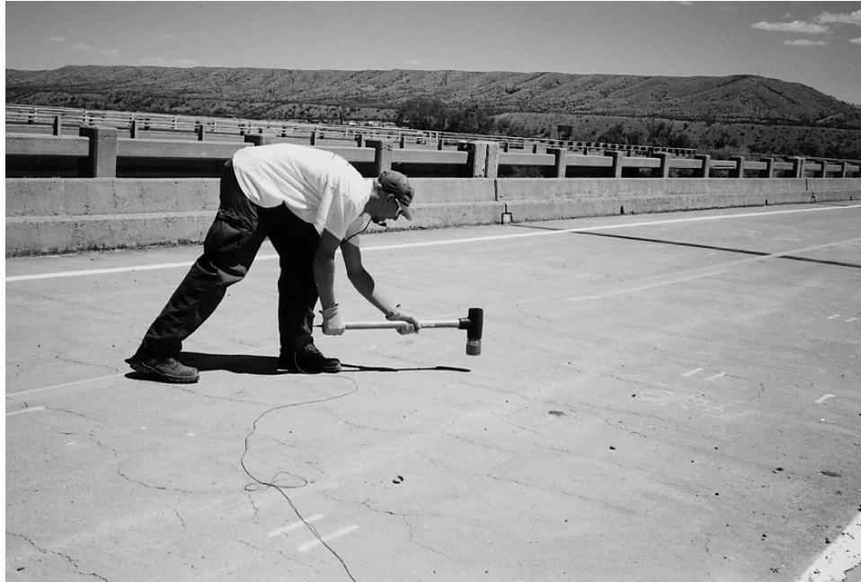
Figure 4-26: Modal hammer used to deliver an impact force to the bridge deck
