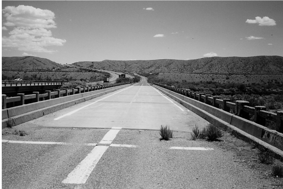
Figure 4-22: Southward top view of the Alamosa Canyon Bridge
