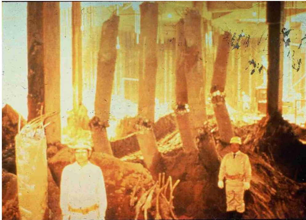
Figure 1.2: Liquefaction-induced lateral spreading effects on piles, 1964 Niigata, Japan Earthquake (Hamada 1991).
