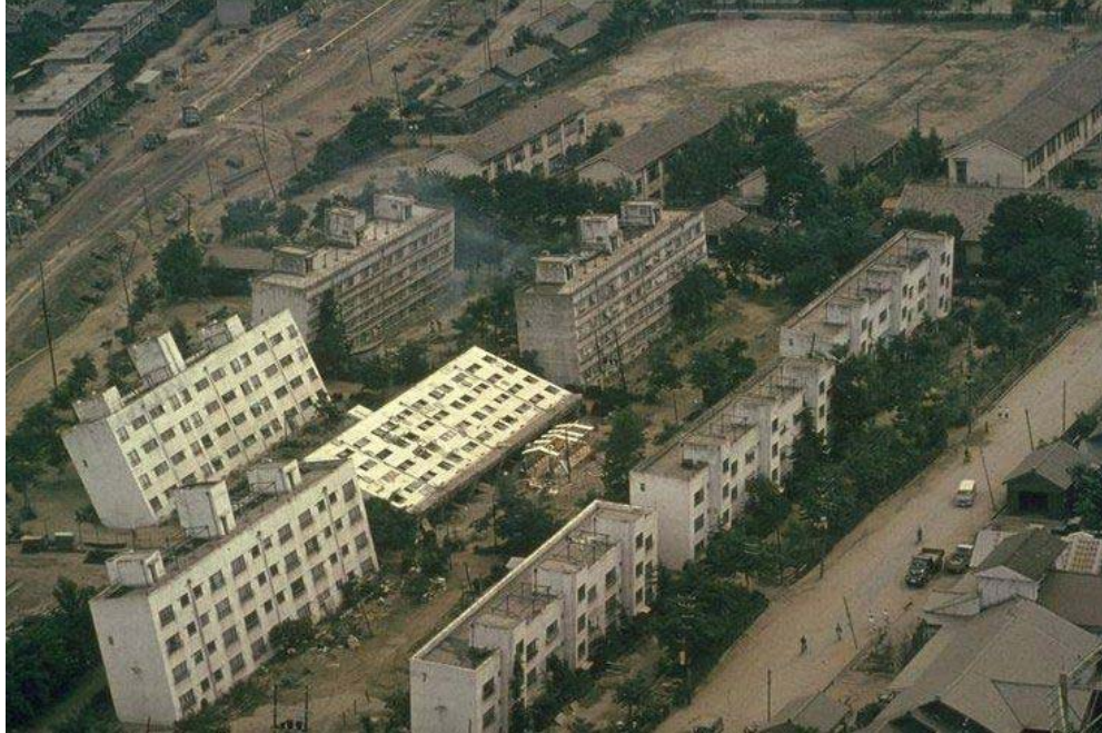
Figure 1.1: Tipped buildings caused by liquefaction-induced loss of bearing strength, 1964 Niigata, Japan Earthquake (Kramer 1996).
