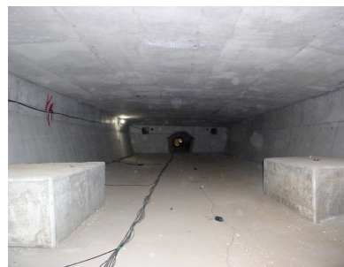
(c) Box girder interior
